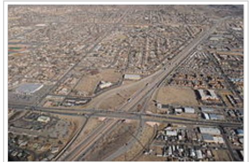
Aerial view of Interstate 40
