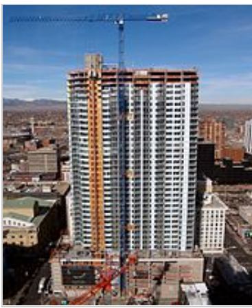
Construction of the Spire, a new 41 story residential building near the convention center
