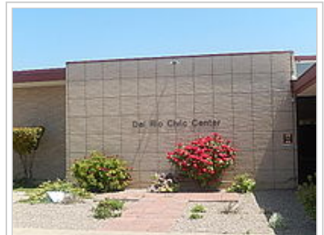
Del Rio Civic Center at 1915 Veterans Blvd.
