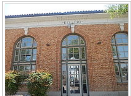
Del Rio Amtrak station
