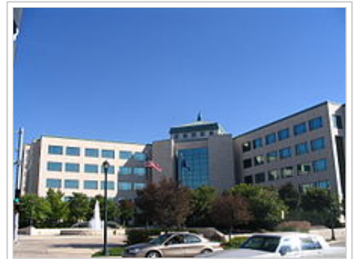
The Charles Curtis State Office Building (2001), facing the capitol
