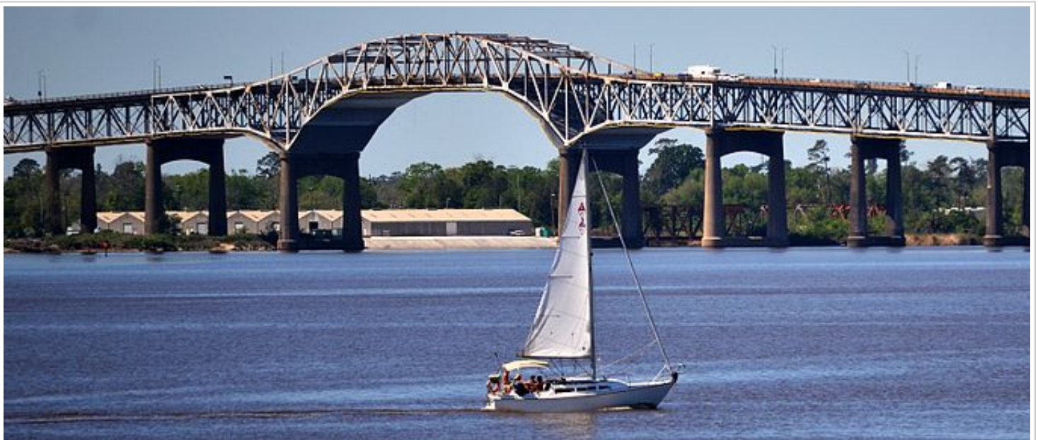
Interstate 10 crossing the Calcasieu River Bridge between Lake Charles and Westlake
