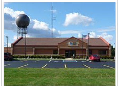
US National Weather Service office, just south of town
