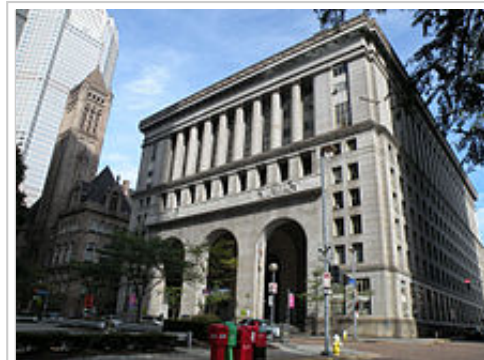
The Pittsburgh City-County Building at right, with the Allegheny County Courthouse at left
