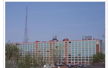
The Larkin Terminal Warehouse, headquarters of First Niagara Bank
