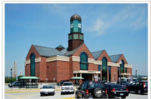
Albany-Rensselaer Amtrak Station
