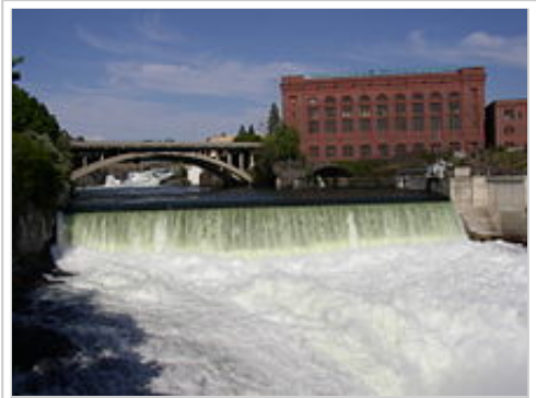
Monroe Street Dam
