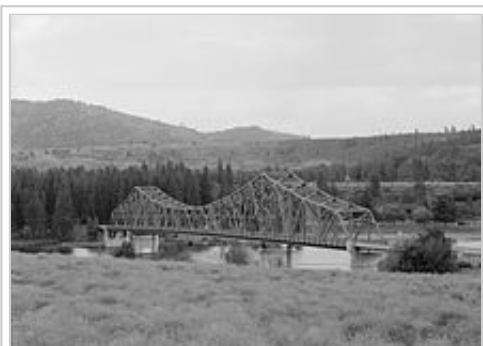
The Spokane River Bridge at Fort Spokane
