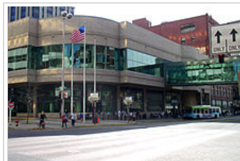
The STA Plaza in downtown Spokane
