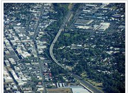
The I-5 viaduct in downtown Medford
