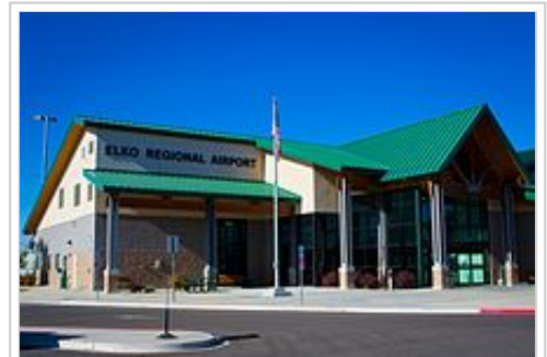
Elko Airport terminal
