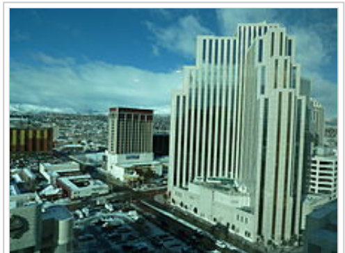
Another view of Reno's highrises with the hotel skyscraper of Silver Legacy
