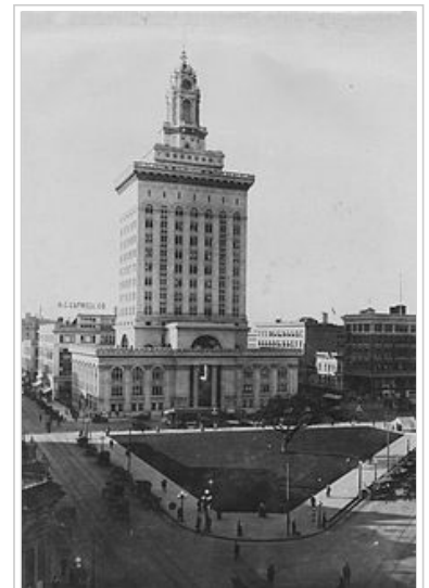
Oakland City Hall and central plaza in 1917. Built of framed steel with unreinforced masonry infill at a cost of $2 million in 1914, the structure was the tallest building in Oakland until the Tribune Tower was built in 1923.
