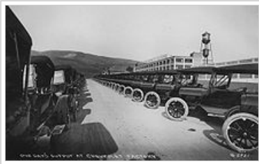
One day's output of 1917 Chevrolet automobiles at their major West Coast plant, now the location of Eastmont Town Center
