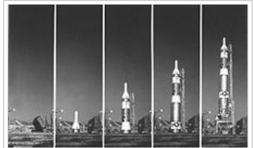
Titan I missile emerges from its silo at Vandenberg Operational System Test Facility in 1960
