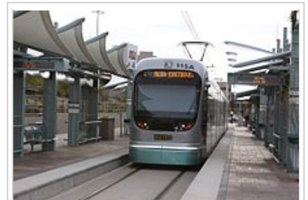
Phoenix light rail station – 2009
