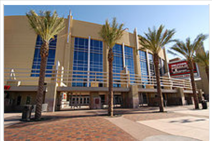
Gila River Arena in Glendale
