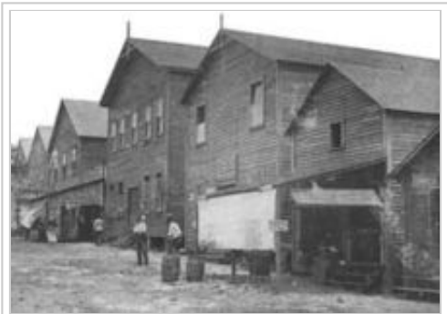
Approximately 400 men voted for Miami's incorporation in 1896 in the building to the left.
