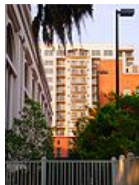
Tennyson Condominiums as seen through a break in the downtown Federal Courthouse Square.
