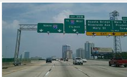
I-95 going through downtown Jacksonville
