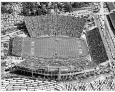
The Gator Bowl Stadium where the annual Gator Bowl has taken place since 1946. EverBank Field now stands on the former site of the stadium which was demolished in 1994.
