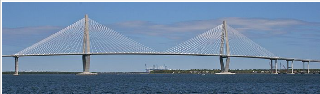
The new Arthur Ravenel, Jr. Bridge, constructed in 2005 and named for former U.S. Representative Arthur Ravenel, Jr., who pushed the project to fruition, was at the time of its construction the second longest cable-stayed bridge in the Western Hemisphere.
