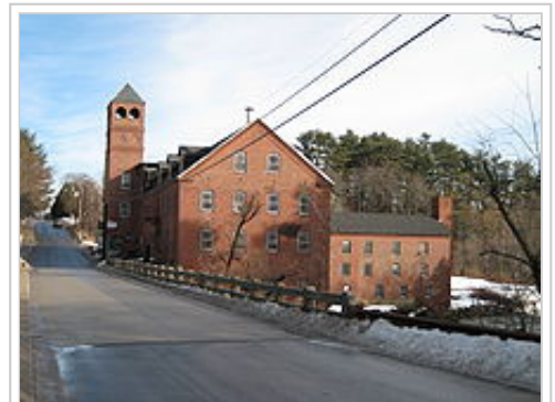
An old cotton mill, Sparhawk Mill, on Bridge Street, is now home to several small businesses. The original structure was built in the 1840s, but was rebuilt after a fire.
