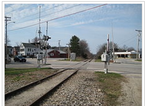
Yarmouth Crossing, where Main Street traverses the St. Lawrence and Atlantic Railroad, looking north.
