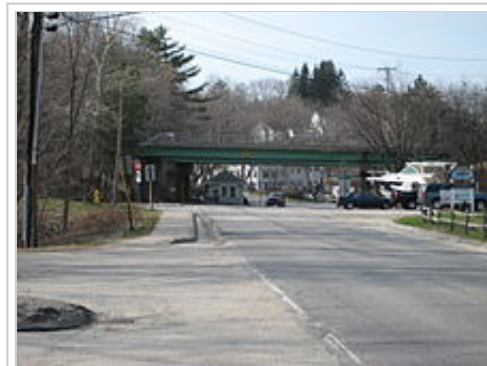
The I-295 overpass on Lafayette Street (State Route 88).
