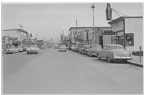
Fourth Avenue in 1953, looking east from near I Street. Just ten years before, the area in the foreground was mostly home to lumber yards and other light industrial uses.
