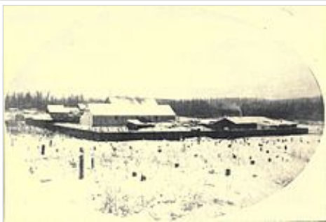
The fledgling settlement of Fairbanks as it appeared in 1903. The buildings shown are likely those of E. T. Barnette's trading post.
