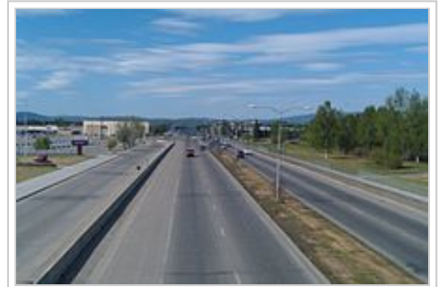
Airport Way (shown at top, eastbound, and above, westbound, from the pedestrian crossing next to Lathrop High School), is the main east-west thoroughfare in Fairbanks. Constructed in the early and mid-1970s, it links the main gate of Fort Wainwright with the main terminal of Fairbanks International Airport.
