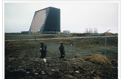
Security policemen patrol the area around the Cobra Dane radar system operated by the 16th Surveillance Squadron. (Older AN/FPS-17 radar antennas appear in the background)
