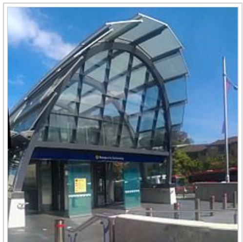
Macquarie University railway station
