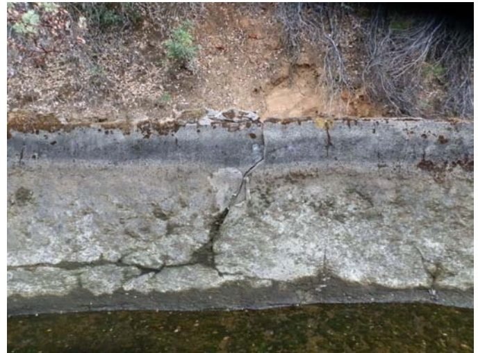
A section of Miner's Ranch Canal prior to restoration
