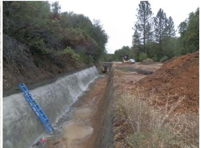
Finished section of Miner's Ranch Canal
