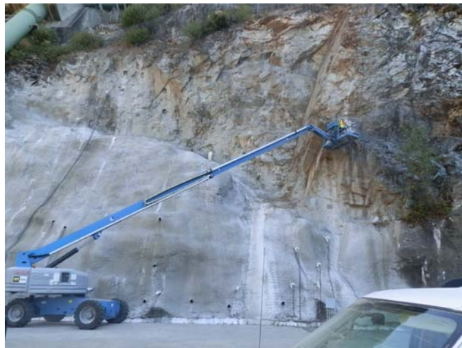
Inspection of Woodleaf Powerhouse Rock slope
