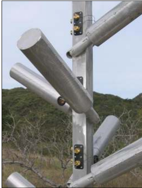
Figure 5.7 Close-up photo of spark arrestors
