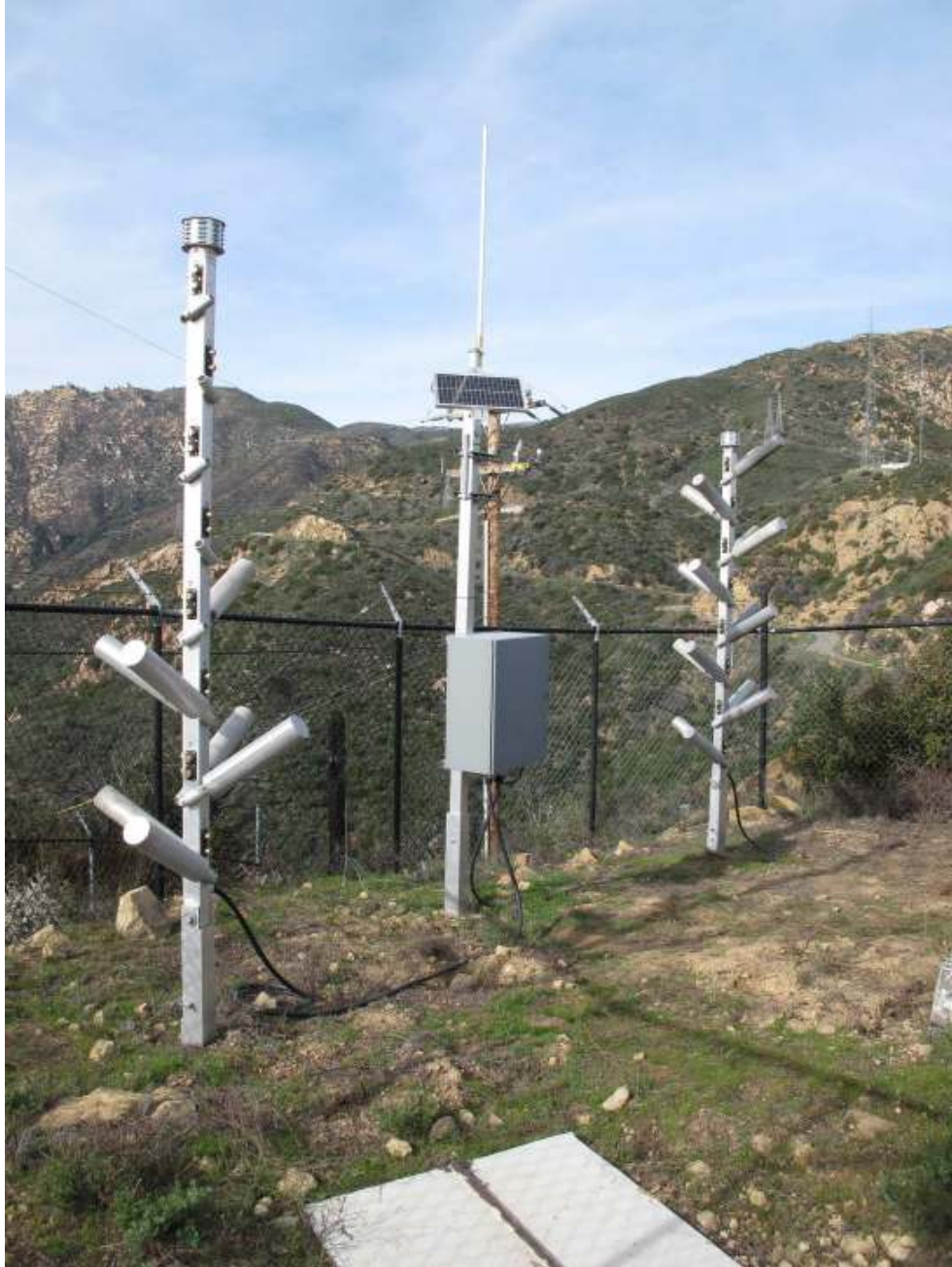
Figure 5.6 Photo of the Gibraltar Road AHOGS site
