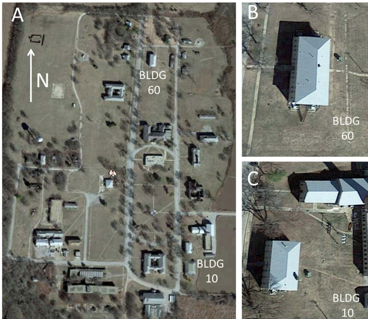
Figure 5. Satellite images of the Chilocco Campus highlighting the location of apartment buildings (A) building 60 and (B) building 10.
