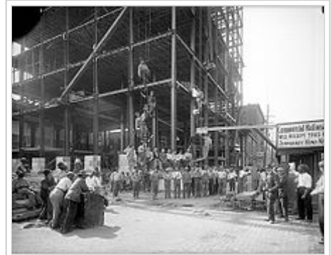
Construction of the Commercial National Bank building, c.1912
