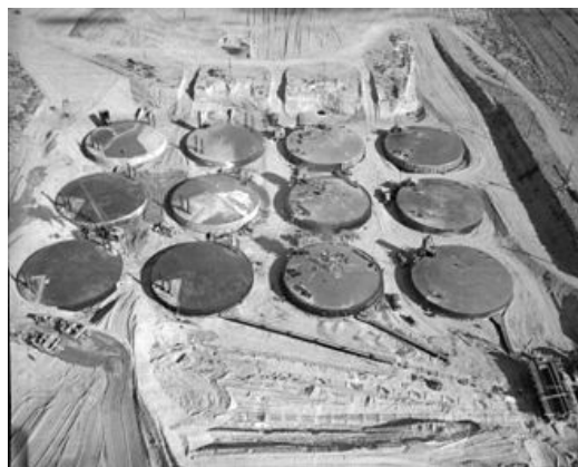
Underground tank farm with 12 of the site's 177 waste storage tanks
