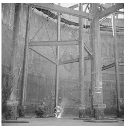
Inside one of the waste storage tanks
