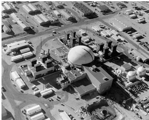
The Fast Flux Test Facility
