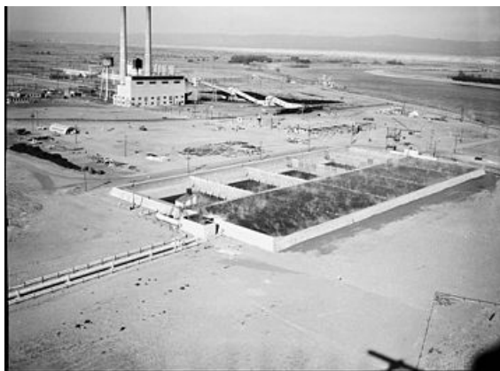
Cooling water retention basins at the F-Reactor
