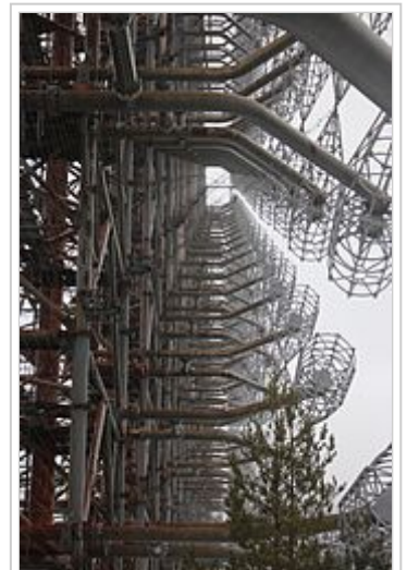
Steel structure of Duga-1 from the bottom
