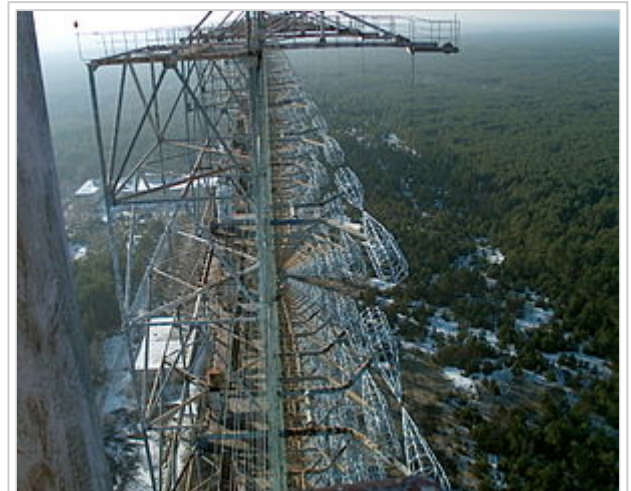
Duga-1 array within the Chernobyl Exclusion Zone. The array of pairs of cylindrical/conical cages on the right are the driven elements, fed at the facing points with a form of ladder line suspended from stand-off platforms at top right. A backplane axial reflector of small wires can just be seen left of center, most clearly at the bottom of the image.
