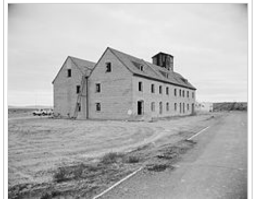
German village in 1994, oblique angle. The roof construction was added in the 1960s
